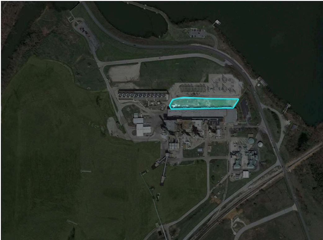
Approximate location of transformers
